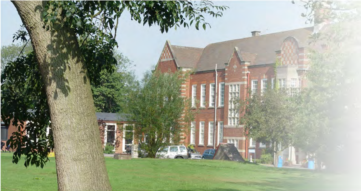
New Infill Administration Offices And Toilet Refurbishment At Wolverhampton Girls' High School
