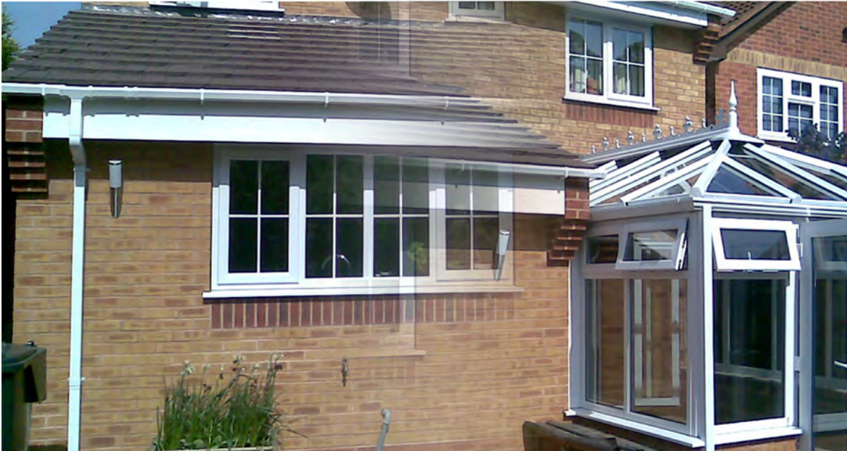
Refurbishment And Extension To An Existing Dwelling In Bromsgrove, Worcestershire
